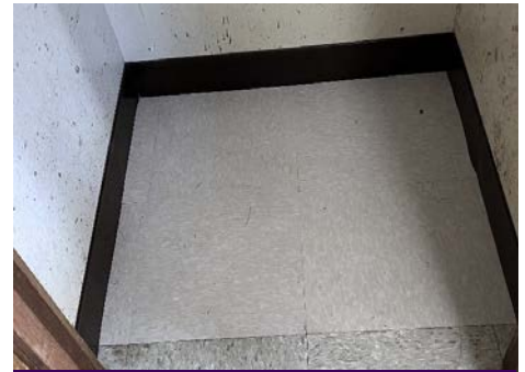
AFTER: Vinyl floor and baseboard installed in the kitchen broom closet.
